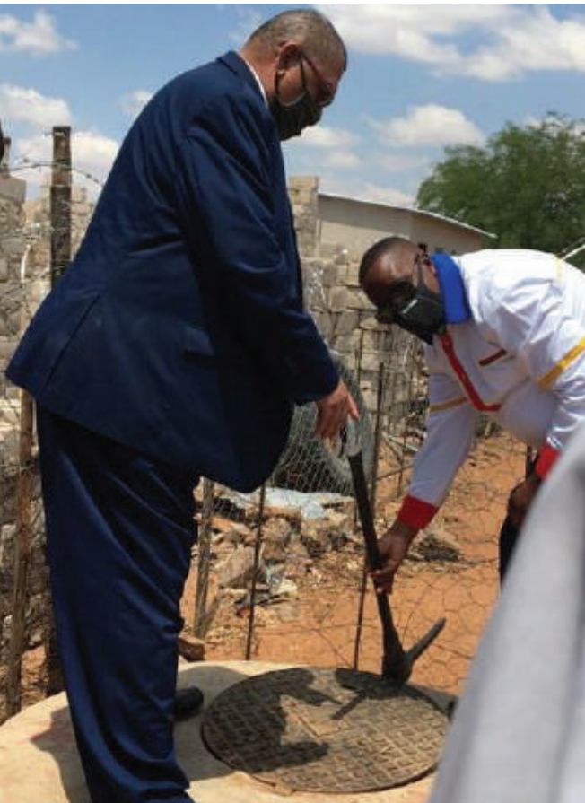
October 2020: Deputy Minister Derek Klazen and Governor Pijoo Nganate officially launched service installations (water and sewer) for 1,115 households in Freedom Square, Gobabis.
